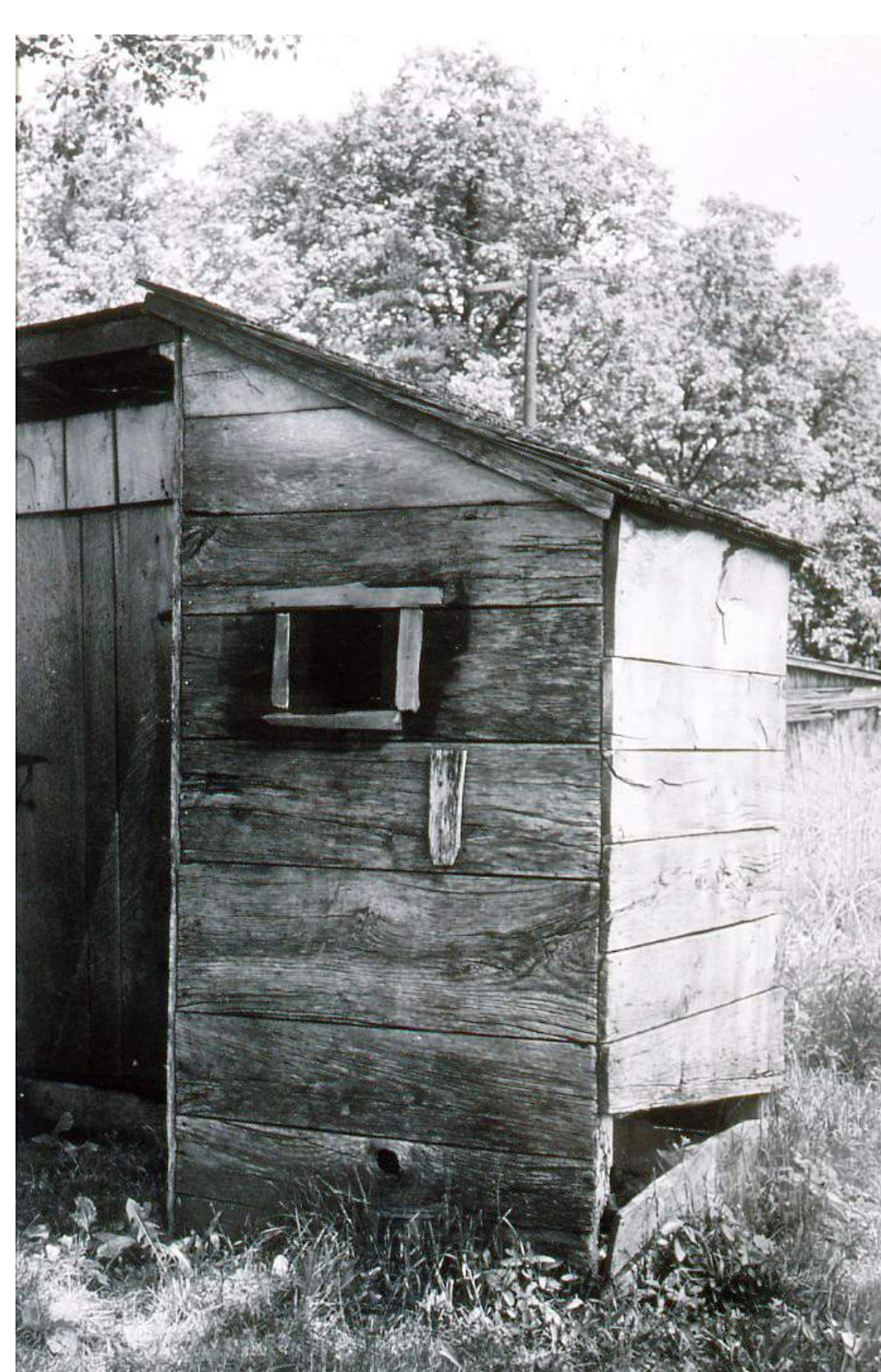
Environmental health, sanitary spring, Montgomery County, Maryland, 1930
