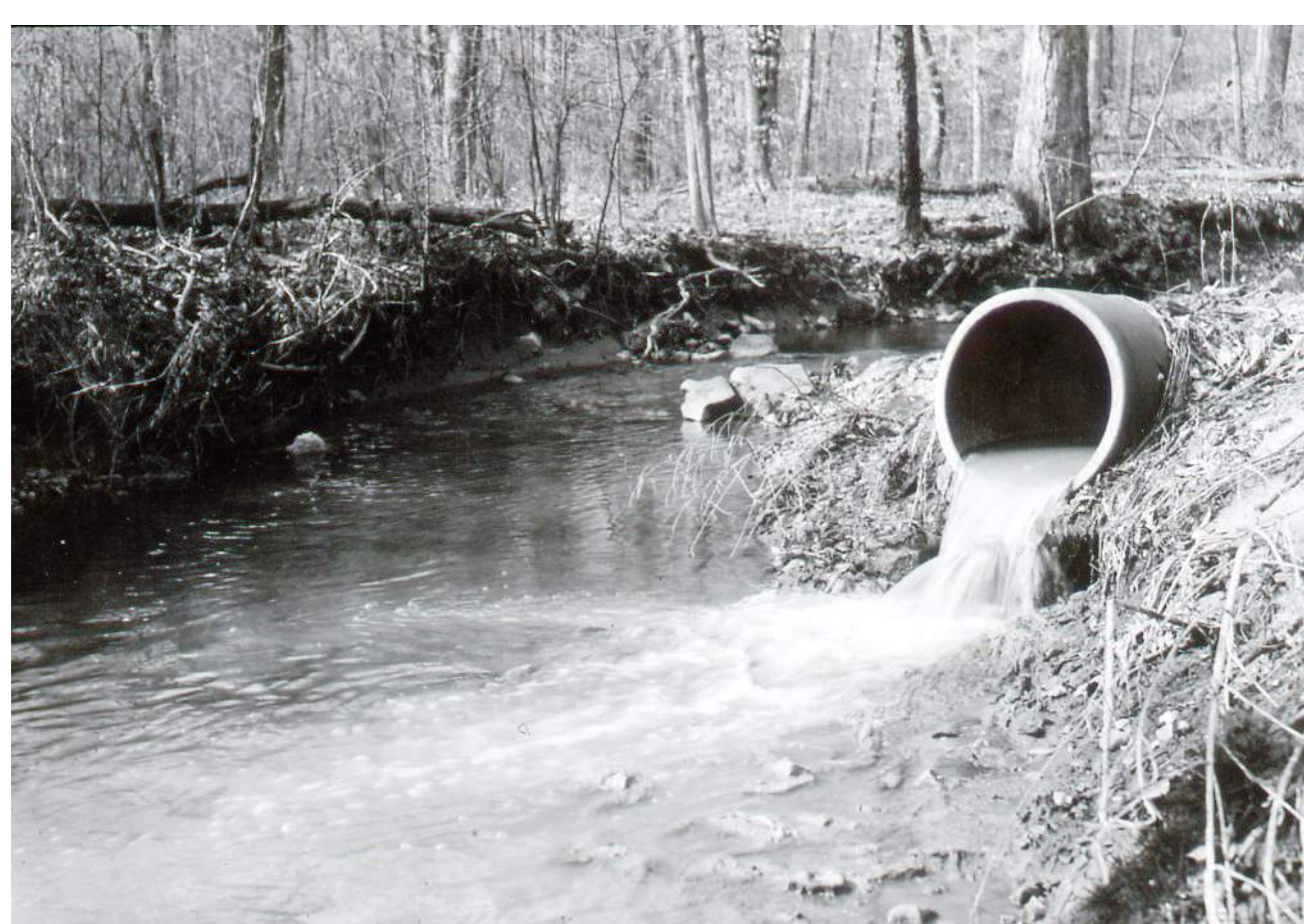
Environmental health, open sewage, Montgomery County, Maryland, 1930s
